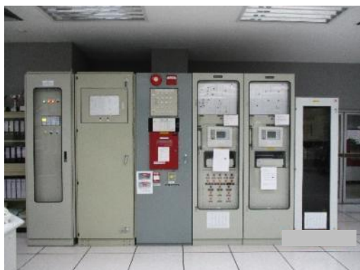
Master Fire Alarm Control Panel
