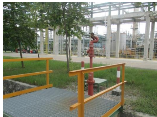
Water Hydrant with Monitor
