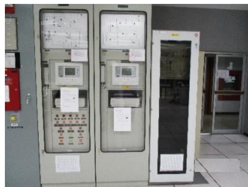
Slave Fire Alarm Panel
